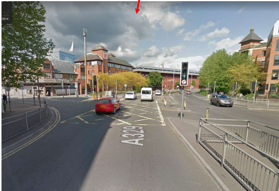
Existing yellow box markings
