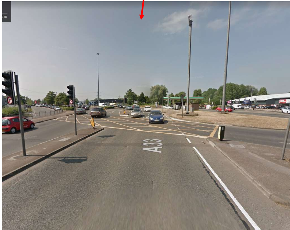
Existing Yellow box markings
