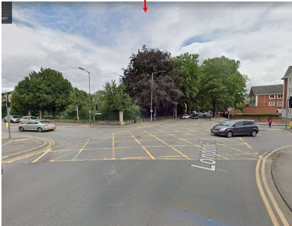
Existing yellow box markings
