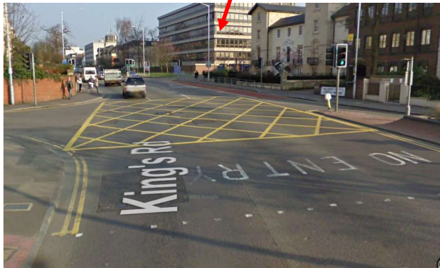
Existing Yellow box markings (A) Kings Road jun Ords Road
