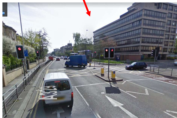
Existing yellow box markings (B) Kings Road jun Eldon Road
